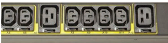
Figure 1. Rack PDUs with IEC outlet grips can reduce the risk of plugs getting bumped loose and leading to server shutdown.
